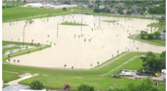
A south Tulsa stormwater detention facility shown storing floodwaters during the May 5, 2000 flooding.
