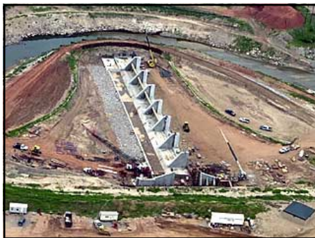
The Oklahoma River was diverted at three locations for construction of low water dams.
